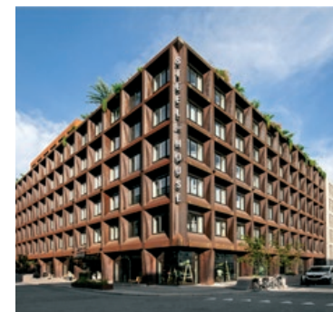
Steel House Copenhagen
